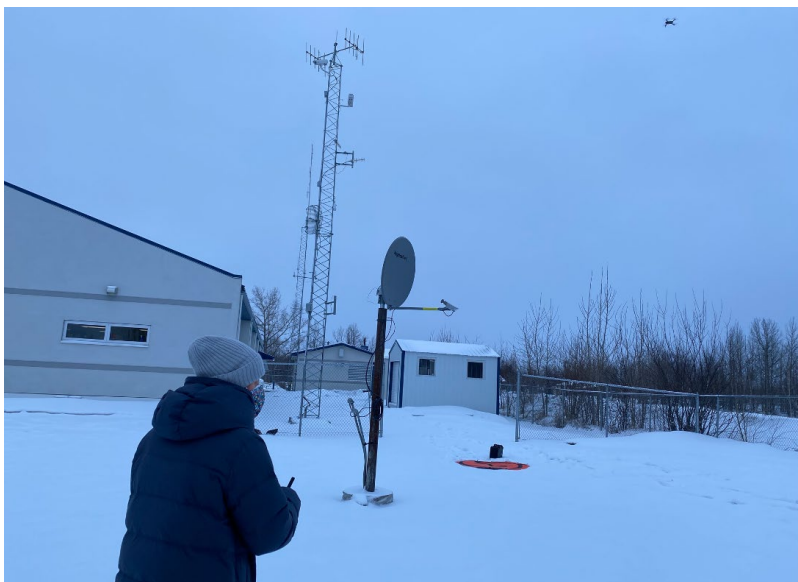
Image 17: At the National Tsunami Warning Center in Palmer, Alaska, a pilot uses a small UAS to inspect an instrument tower for damage from a mid-winter wind storm. Photo: NESDIS/NOAA
